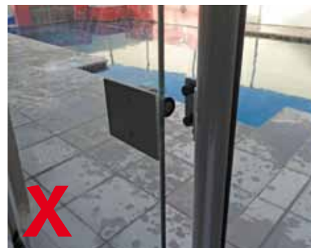
The gate or components may need to be adjusted or replaced to ensure self-closing mechanism works properly.
