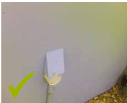
A power outlet has been shielded appropriately.
