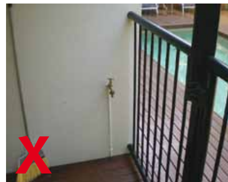
A tap fitting is a climbable object and must be shielded or removed.
