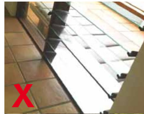
Louvres that create a gap of more than 100 millimetres do not comply.
